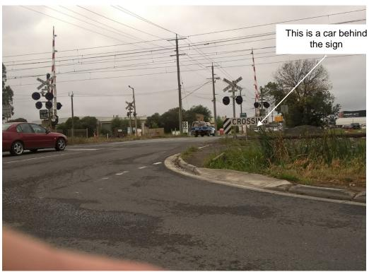
As the sight line issues at this intersection are created by the railway level crossing it is not possible to treat this intersection without altering the railway level crossing, which would be a multi-million dollar project.
