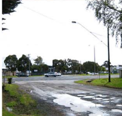
GLISMANN ROAD & PRINCES HIGHWAY EXISTING INTERSECTION
