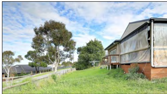
Figure 8: Site visit photo - subject site from Carey Crescent.
