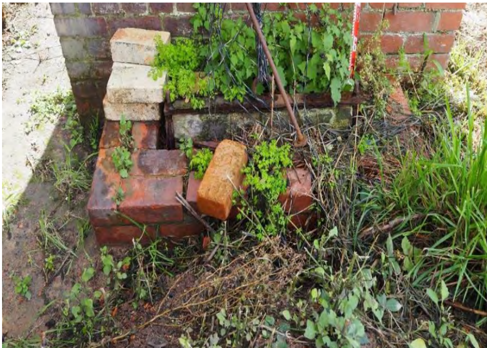
Figure 21 Flue damper on south side of chimney (G. Vines 10/5/2023)
