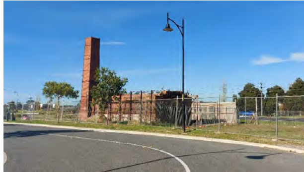
Image: Looking south from Grace Street towards the Subject Site and Princes Highway
