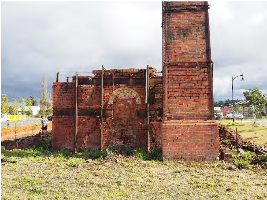
Figure 17 Eastern elevation of kiln showing bricked-up opening (G. Vines 10/5/2023)
