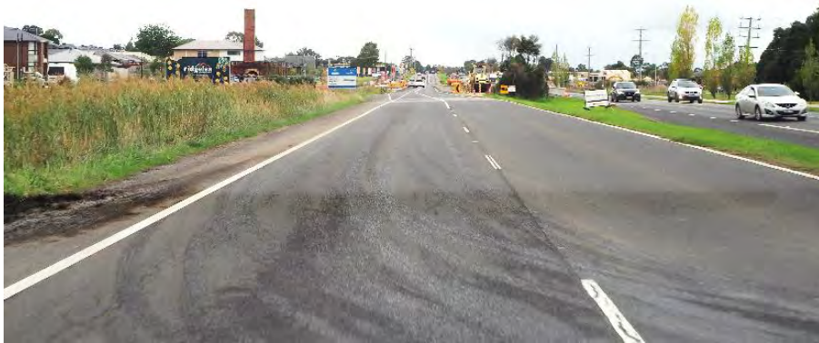
Figure 24 Looking east along Princess Highway with Hicks kiln on right and Berwick Pottery in left distance (G. Vines 10/5/2023)
