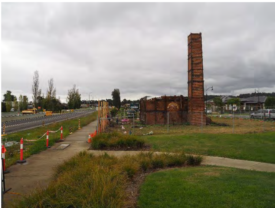
Figure 25 View from small park east of kiln looking west (G. Vines 10/5/2023)
