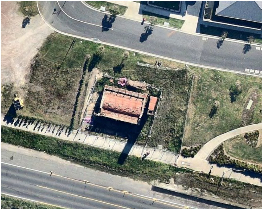
Figure 1 Aerial image from 2023 showing remaining kiln and chimney (NearMap)
