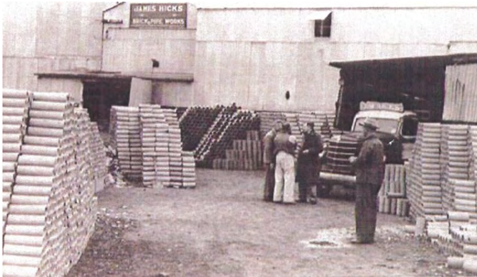
Figure 6 Agricultural drainage pipes stacked in the pottery yard 30
