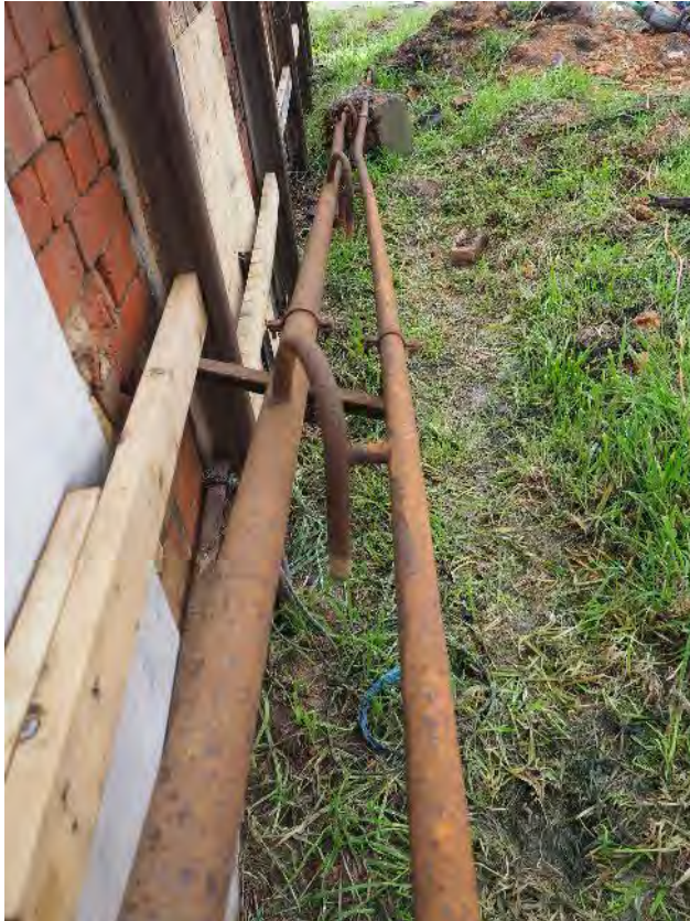
Figure 18 Gas pipes for firing the kiln (G. Vines 10/5/2023)
