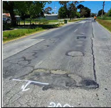
Dalmore Rd - Before Works
