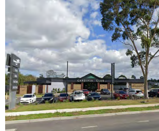
2. CARDINIA CLUB SINGLE STOREY COMMERCIAL BUILDING
