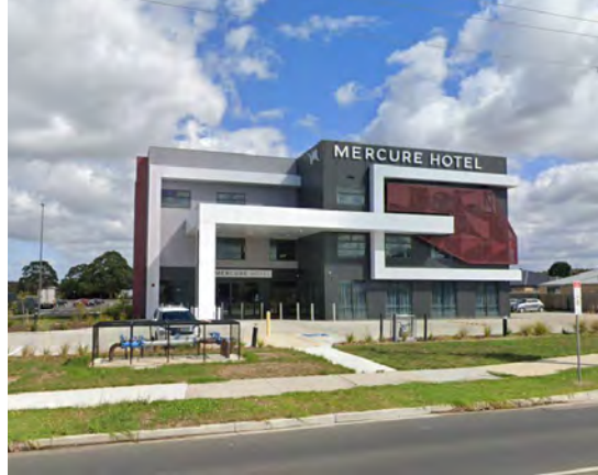
1. MERCURE HOTEL 3 STOREY COMMERCIAL BUILDING
