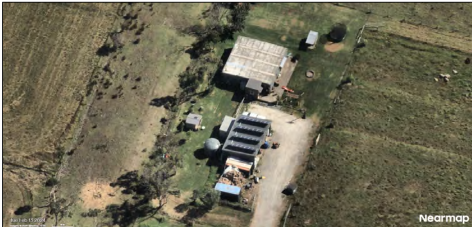
Figure 14: Existing Development - Dwelling (Top) & Shed (Bottom)
