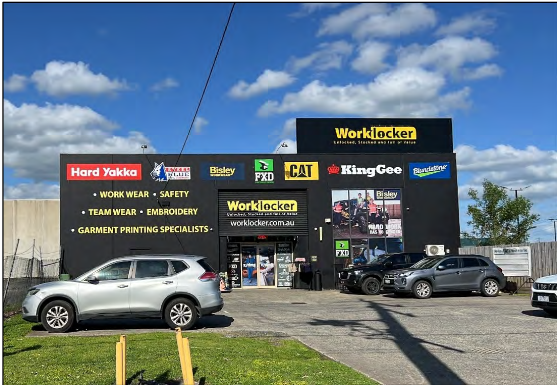
Figure 6 - Existing signage along building frontage (Source: Site Visit 10/08)
