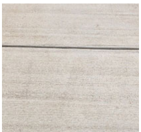
Exterior concrete paving – Broom Finish
