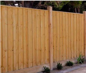
FENCE TYPES 1-3 - FN1, FN2, FN3 DESCRIPTION: ACQUSTIC FENCE TO MEET ACOUSTIC REPORT REQUIREMENTS LOCATION: REAR & SIDE BOUNDARIES
