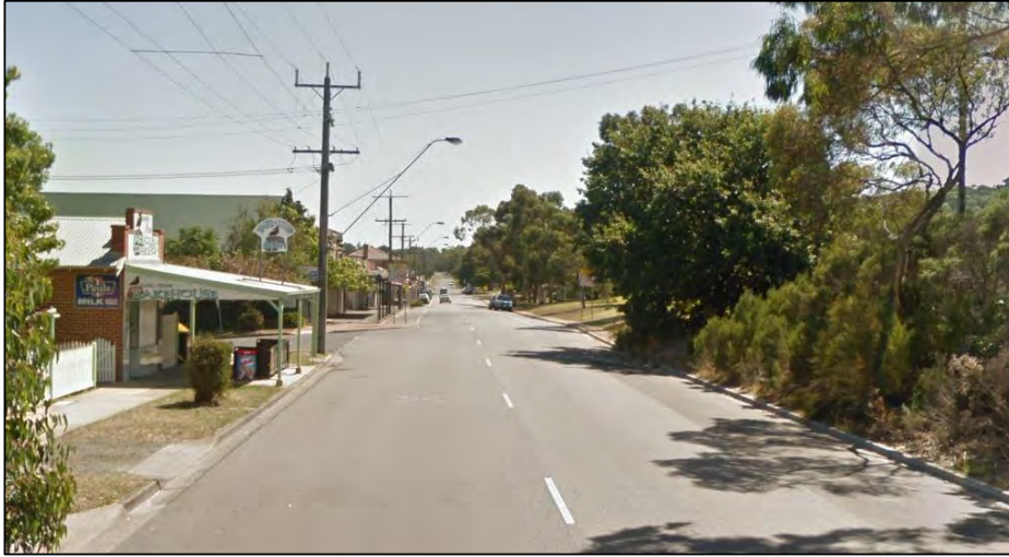
FIGURE 5: NAR NAR GOON-LONGWARRY ROAD FACING NORTH-WEST
