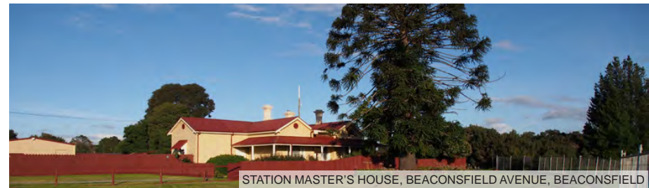
STATION MASTER'S HOUSE, BEACONSFIELD AVENUE, BEACONSFIELD
