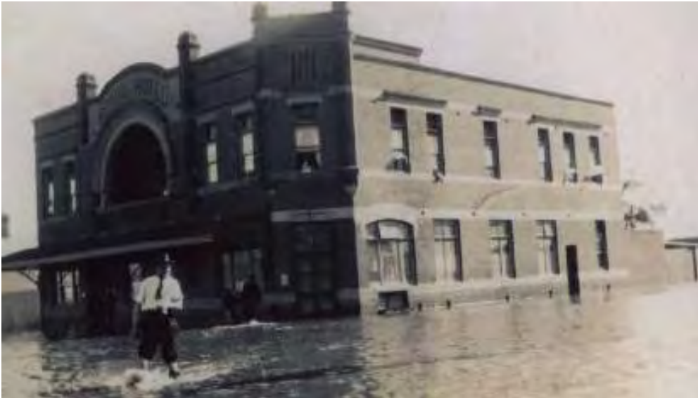
Photograph 11 | Royal Hotel circa 1934 during a great flood of the area
