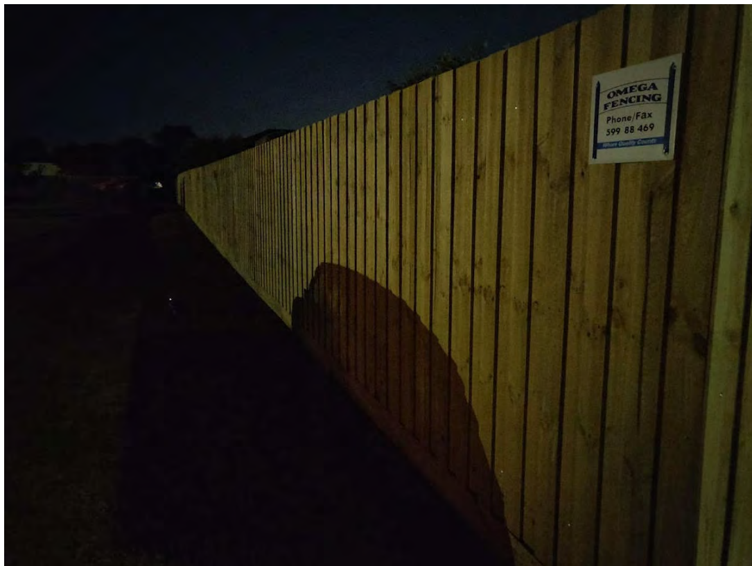
Boundary Fencing to 19 Moody Street and 55 Gardner Street
