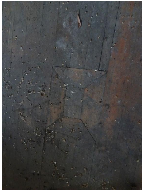
Image 10: Remaining original hardwood floorboard indicating some of the repairs and alterations.
