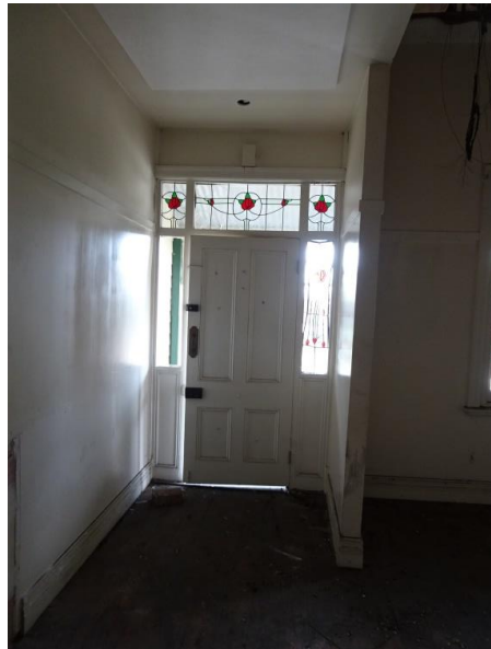
Image 8: Interior of intact front door and trims Note – skirtings and interior linings are of later date
