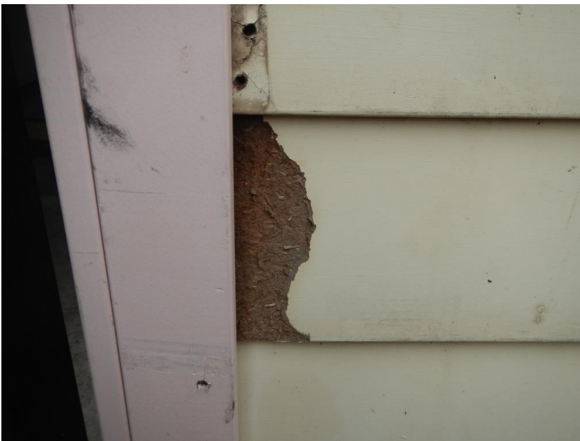
Figure 8 The North side of the Post Office. The cladding is compressed fibre building sheet not weatherboard.
