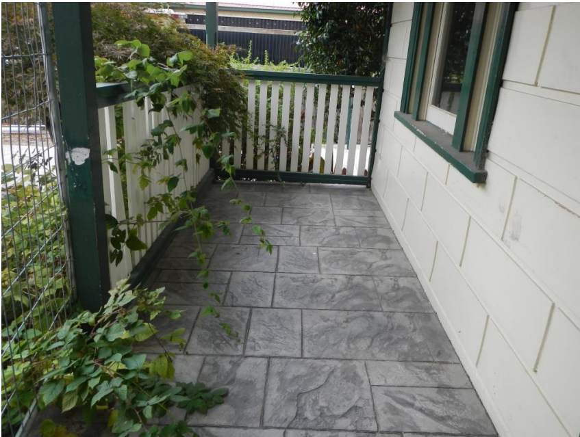
Figure 21 The verandah floor has been paved with faux stone. There may be timber boards beneath.
