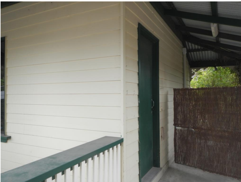
Figure 6 The back of the Post Office. The cladding is building sheet not weatherboard.
