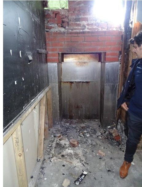
Image 11: Interior view of fireplace which has been relined with modern facebrickwork and st. steel sheeting to comply with modern Health Standards.
