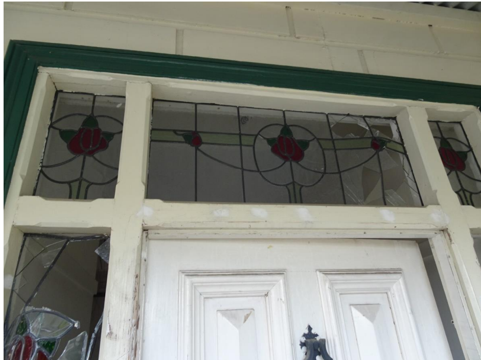
Image 3: The front door and frame complete with leadlight surround (of later date and recently vandalised).
