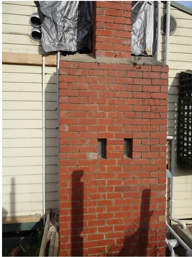
Image 7: The brick chimney remains intact and is in reasonable condition. Note the chimney lights – an important feature of Edwardian fireplace.
