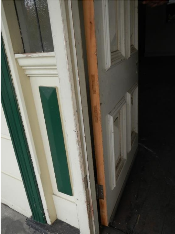
Figure 17 The fact that the door has been cut down lends support to the likelihood that the door is salvage from elsewhere installed as a replacement rather than original otherwise there is no obvious reason as to why it was cut down.
