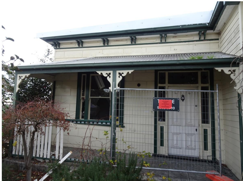
Image 2: The front façade of the c1910 dwelling is good condition and most intact. The verandah is of later date and not architecturally significant.
