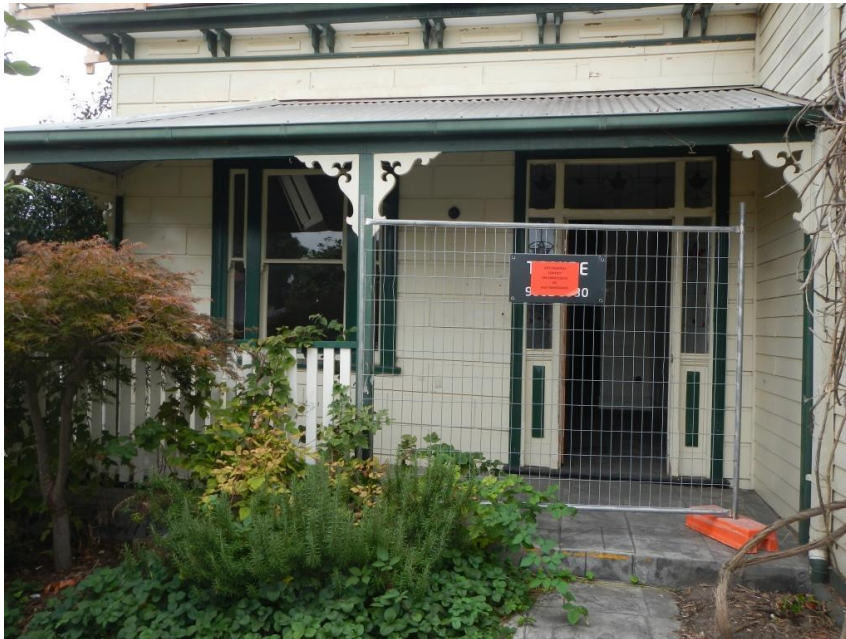
Figure 15 The timber block-fronted façade to the residence.
