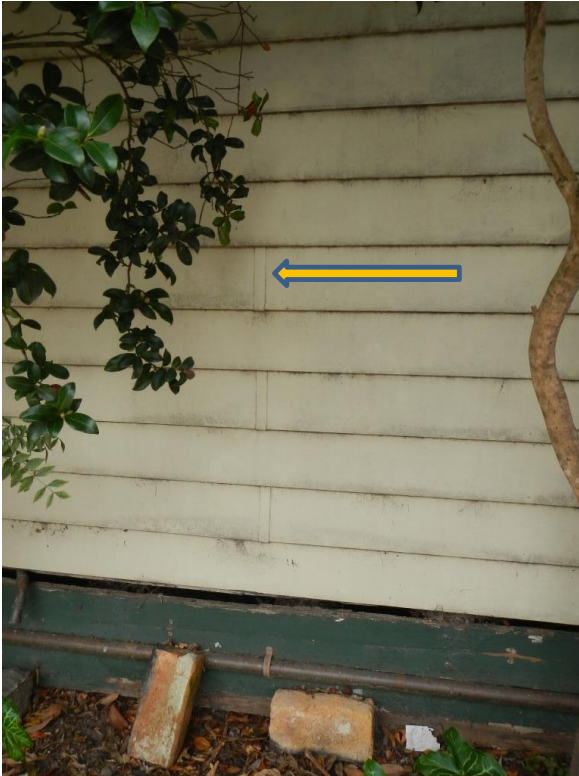
Figure 24 The cladding on the South side is similar to that on the North side of the Post Office and joints have been concealed or fixed with clips. It is not timber weatherboard.
