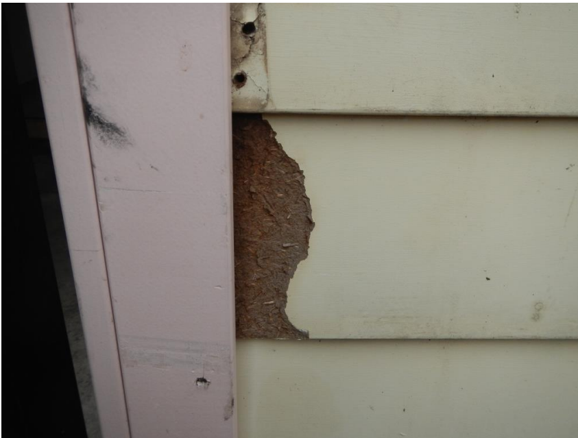
Figure 8 The North side of the Post Office. The cladding is compressed fibre building sheet not weatherboard.
