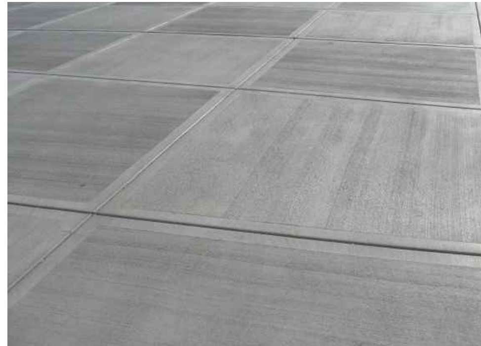
BRUSHED CONCRETE LOCATION: EXTERNAL PAVING
