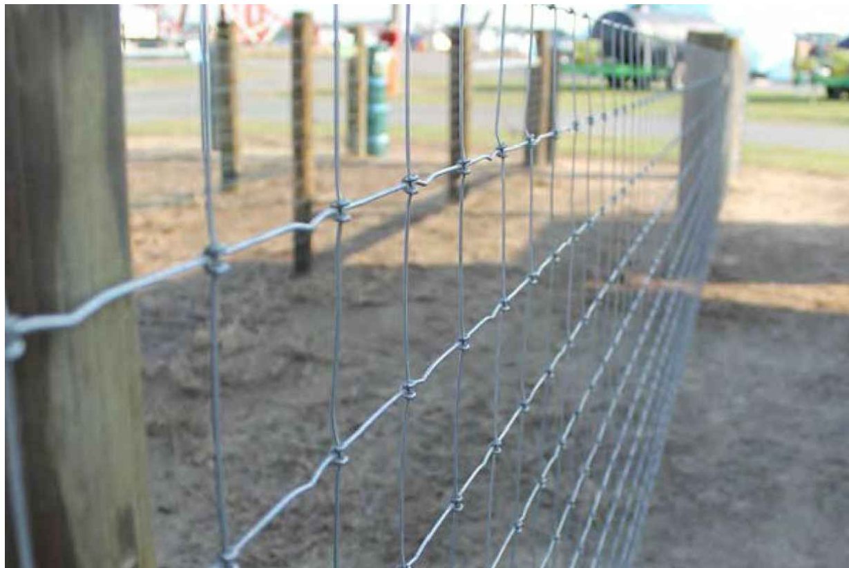
FENCE TYPE FT2 - TIMBER POSTS AND RINGLOCK WIRE FENCING PHOTO
