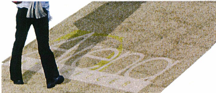
Surface Branding Sand blasted logo/branding on exposed Aggregate concrete surface
