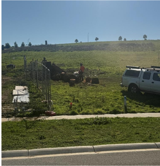
Figure 1. Evidence that the tree removal has been completed
