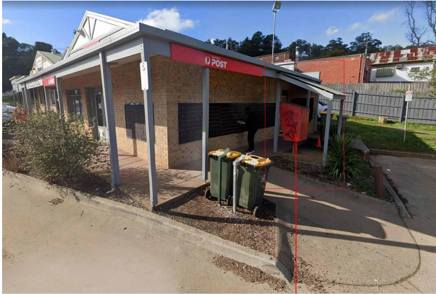
AREA WHERE WORKS IS BEING PROPOSED
