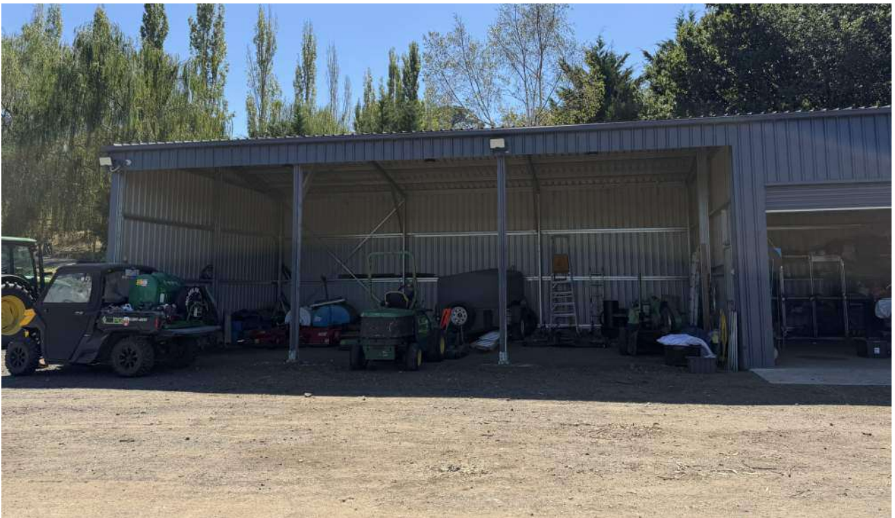
Shed 3 open bays
