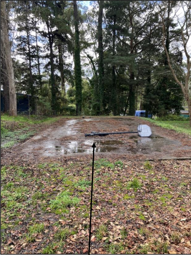
Existing concrete slab
