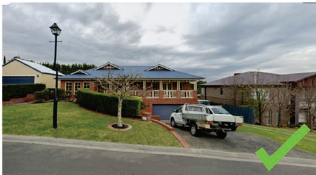
On lots with grades over 10% with side to side fall, driveways on the low side allow for split level design responses that limit retaining walls on boundaries
