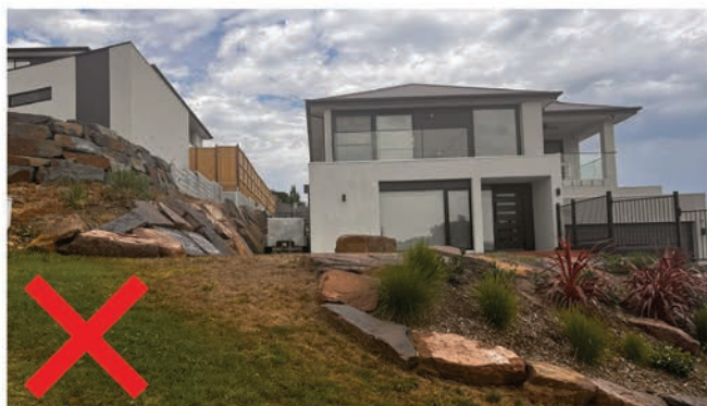
Split level home on lot with side to side grade on pre-development slope in excess of 20% still requires significant cut and fill
