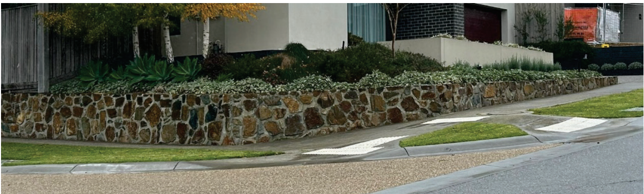
Figure 25 - Rock retaining wall along property street frontage, including along the street corner side boundary
