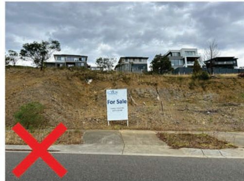
Avoid subdivision of small lots on steep (in excess of 20% grade) land
