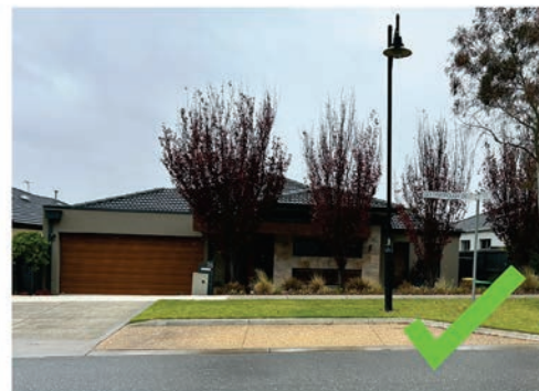
Where lots fall away from the road, ensure the dwelling maintains a street presence and the driveway is a manageable grade
