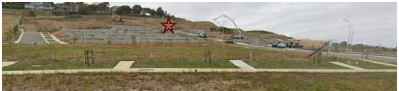
Figure 7 – The Rise Estate under construction (Google Streetview)
