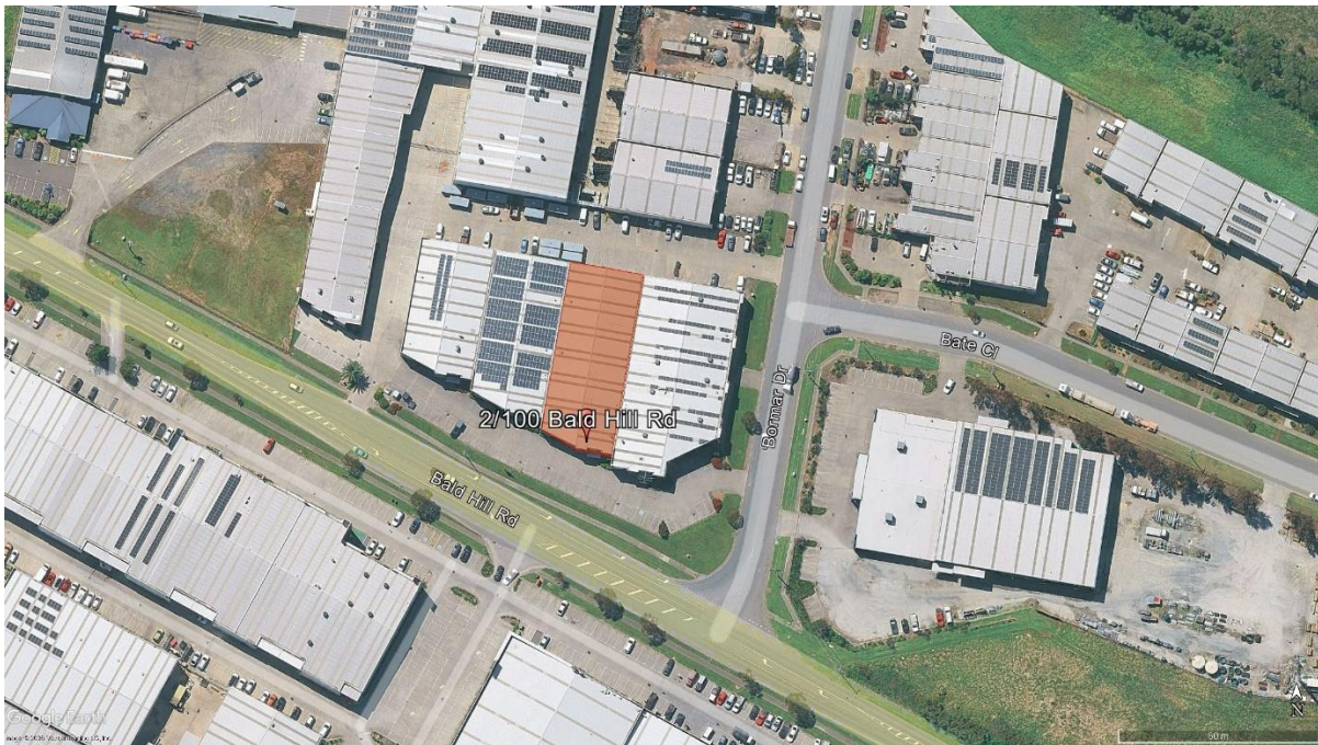
Figure 01; Existing site view of the proposed development
