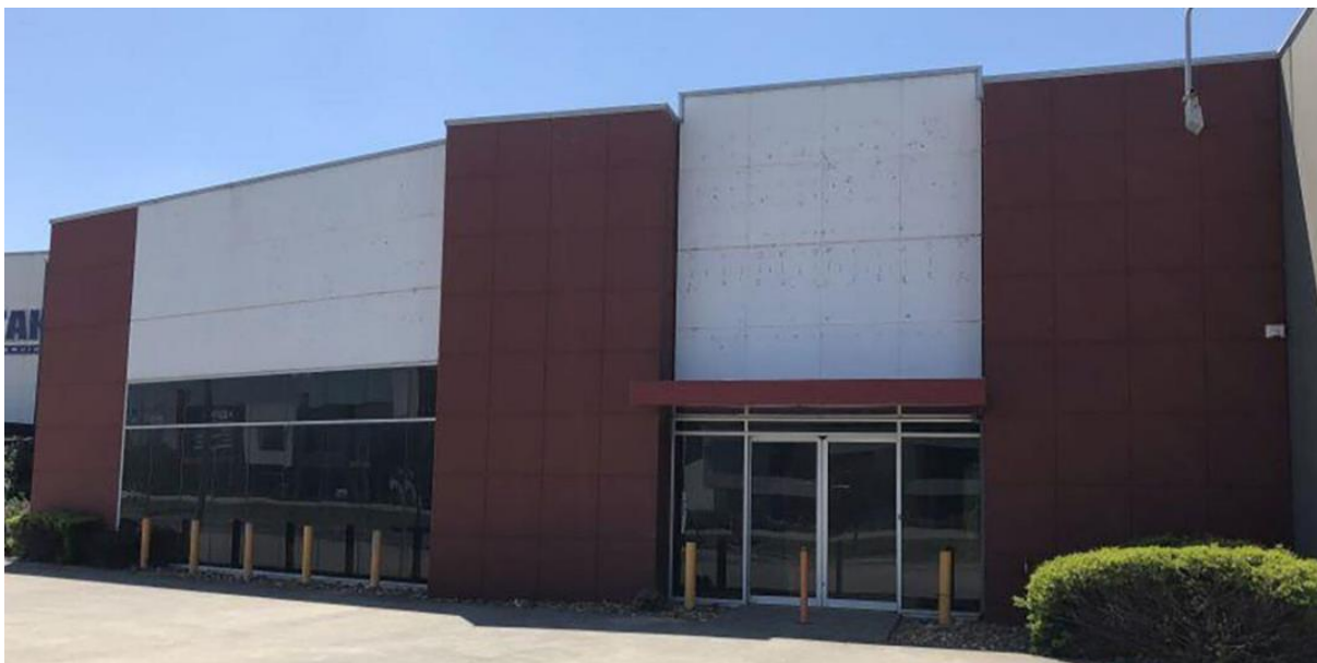
Figure 2: Front façade of the building
