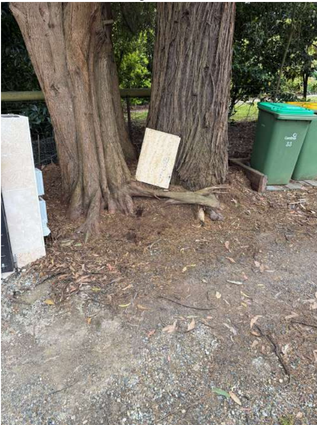
Figure 9: Exposed root structure at base of T1&T2 on driveway
