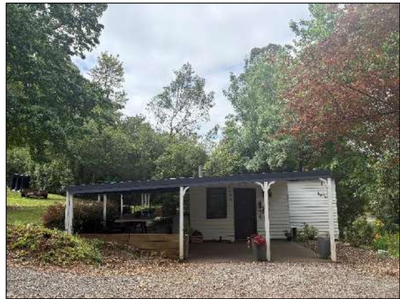
Plate 5 Northern elevation of the subject dwelling
