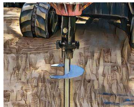
Low impact footings: i.e. - screw piles
