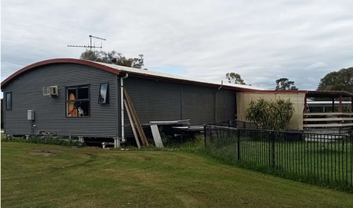
IMAGE 9 – South western view of the existing dwelling.
