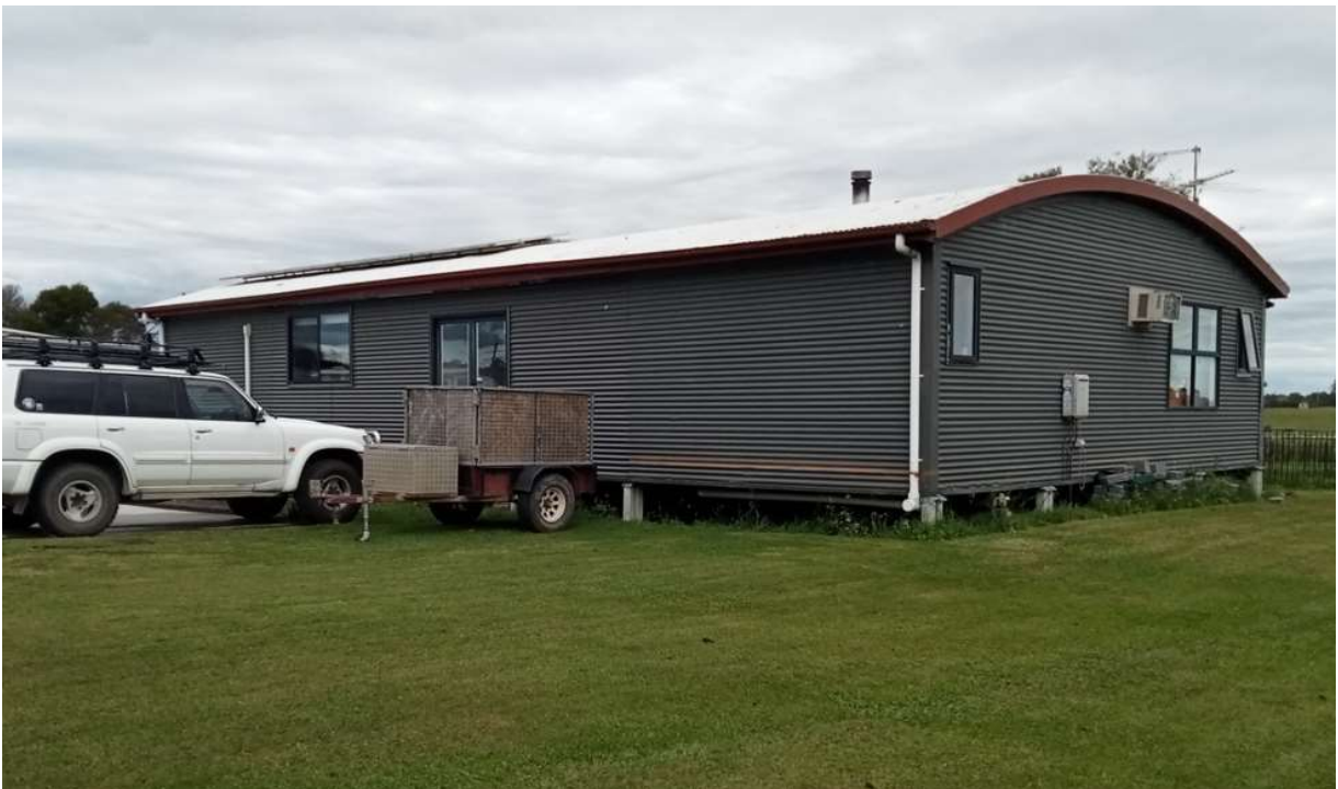
IMAGE 8 - North western view of the existing dwelling.
