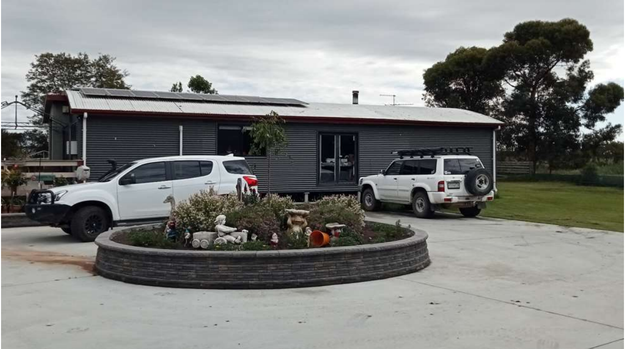
IMAGE 7 – Northern view of the existing dwelling.
