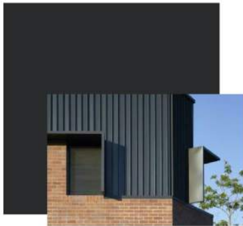
CLM-01 STANDING SEAM MONUMENT CLADDING MONUMENT PROFILES, RFA-01 FLASHINGS & FASCIA, GUTTERS & DP-01 DOWNPIPES
