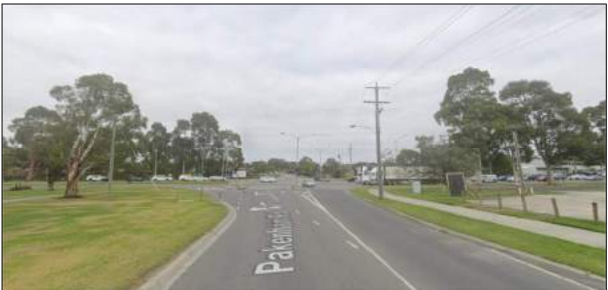
Figure 2.6: View of Pakenham Road facing southwest
