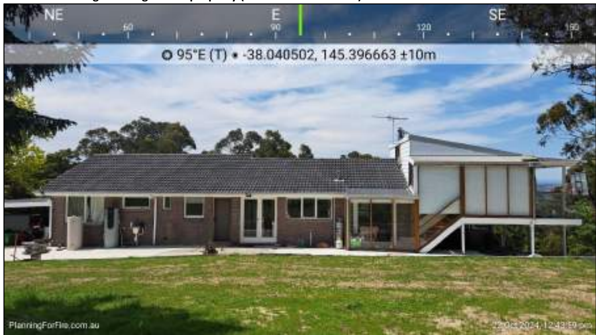
Photo 2 – Existing dwelling on the property (north west elevation)
