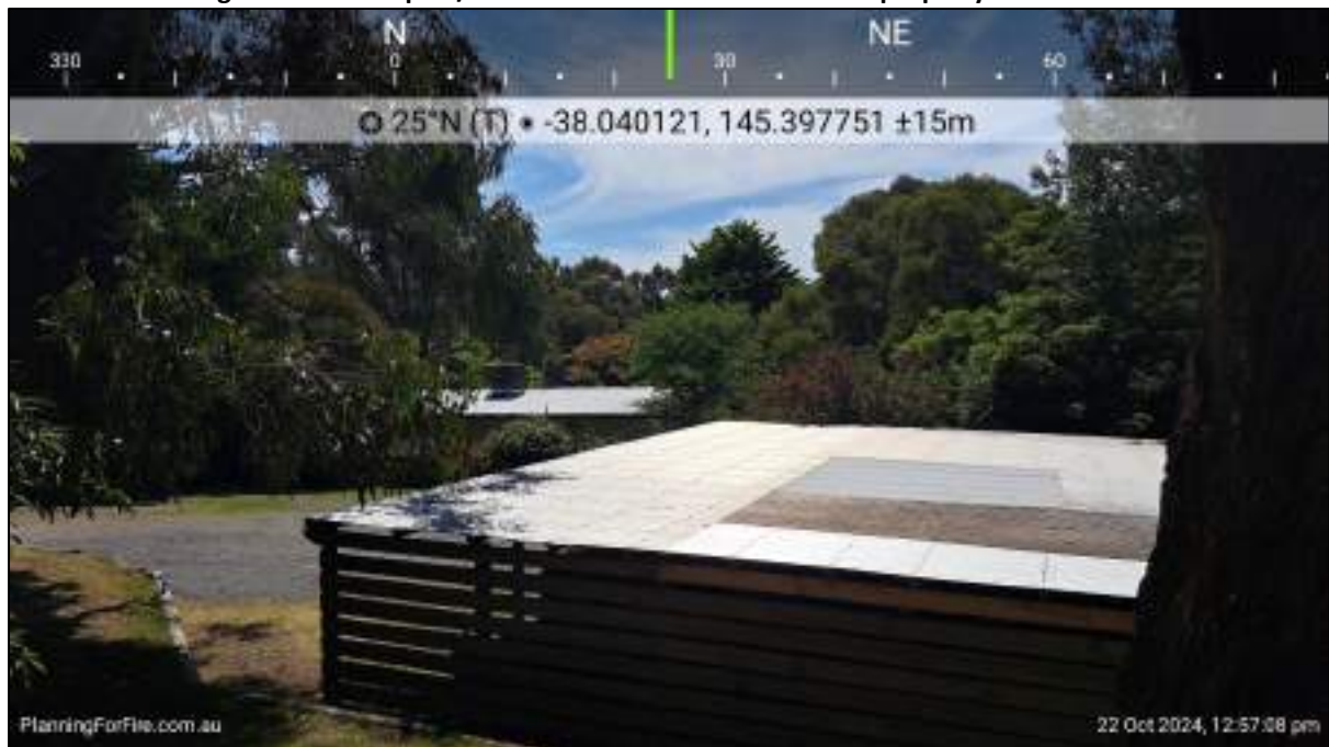
Photo 25 - Looking across the carport/shed at 262 O'Neil Road from the property.
