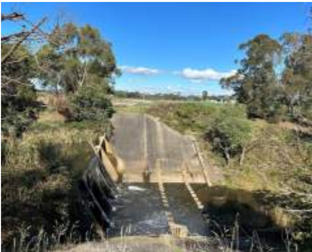
Plate 9 Existing regulator at time of assessment, May 2024
