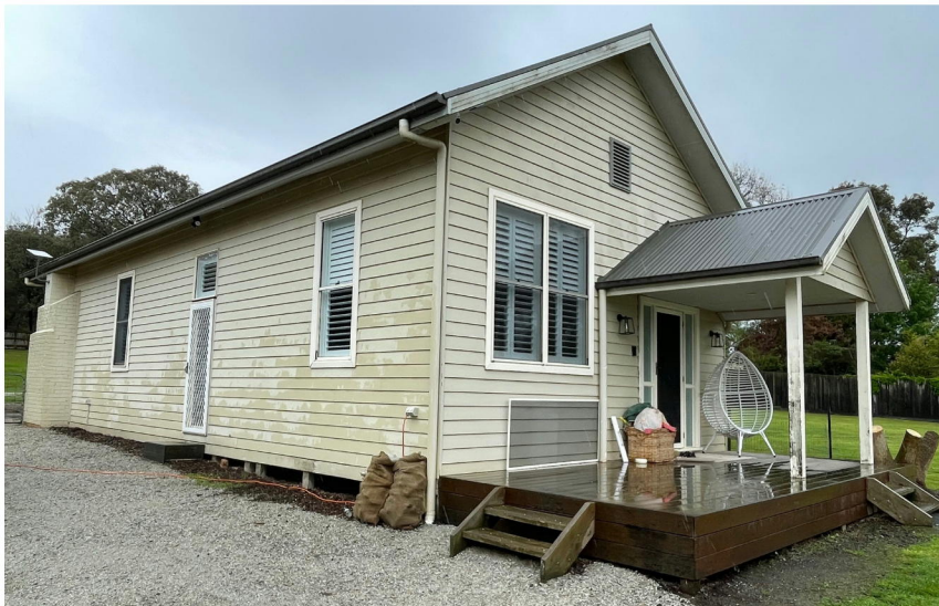
The front of the existing hall.
