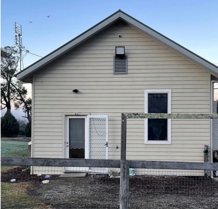
The rear of the existing hall.
