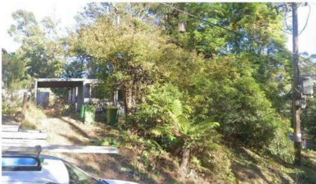
No. 18 Hillside Rd
