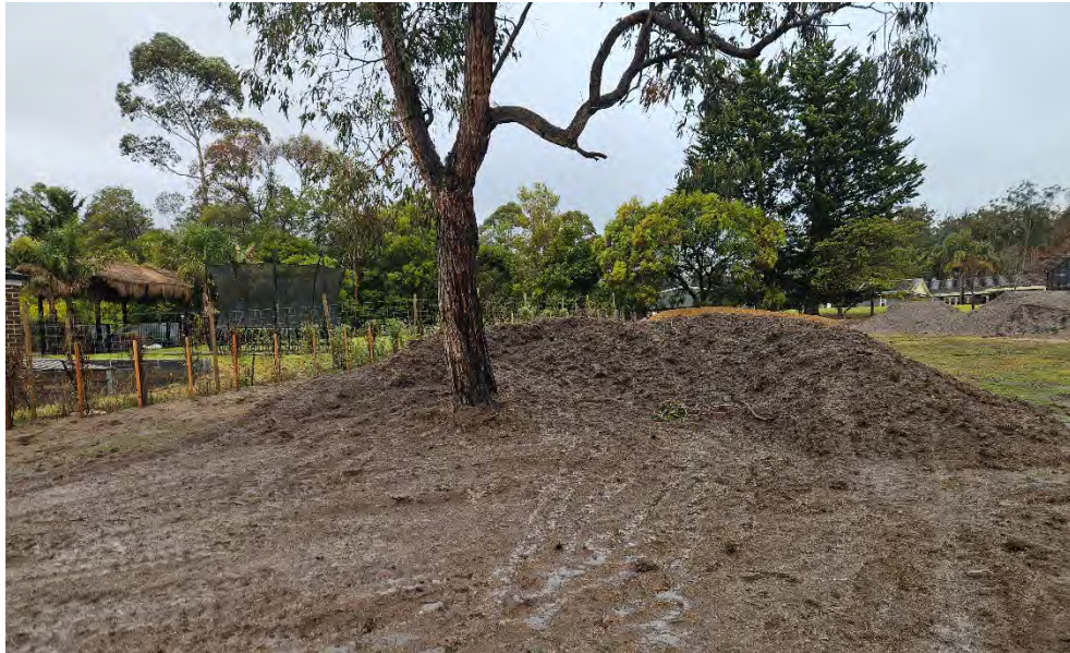
Figure 7: Fill soil within the NRZ of Tree 14
