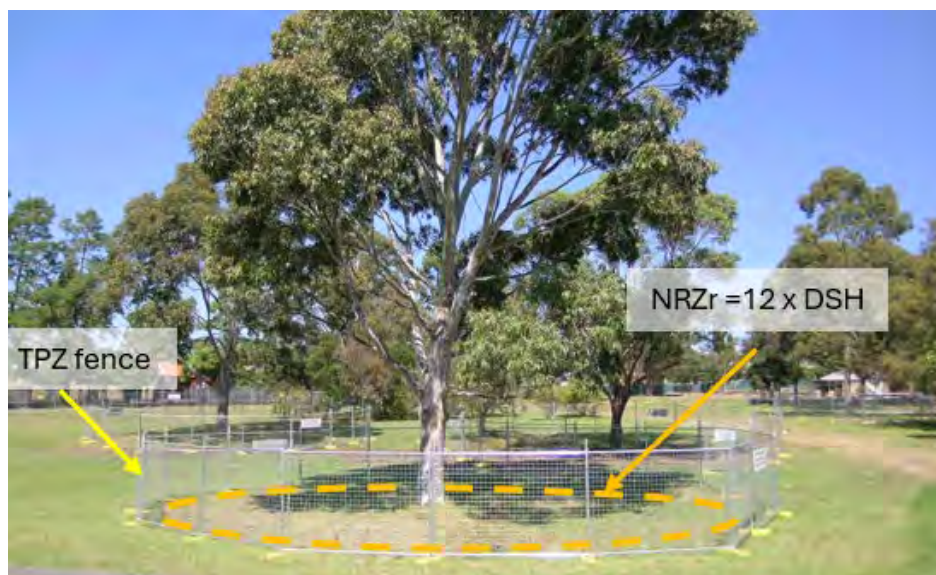
Figure 10: Tree protection fencing is erected around retained trees prior to site works
