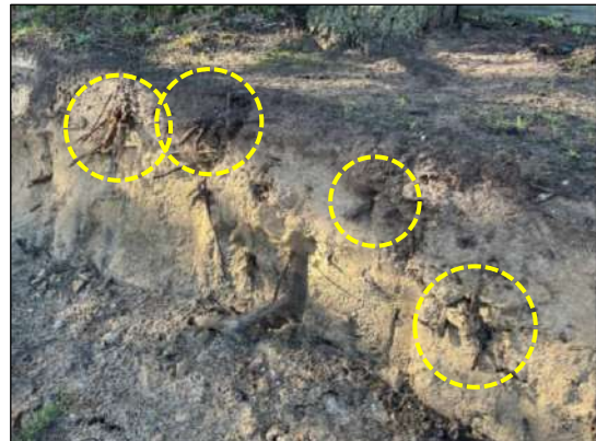
Plate 1 – Showing root severance to Tree 1 from the recent site cut.
