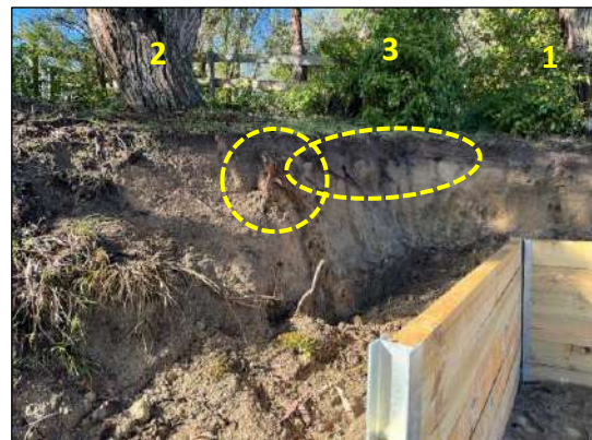
Plate 2 – Showing root severance to Tree 2 from the recent site cut.
