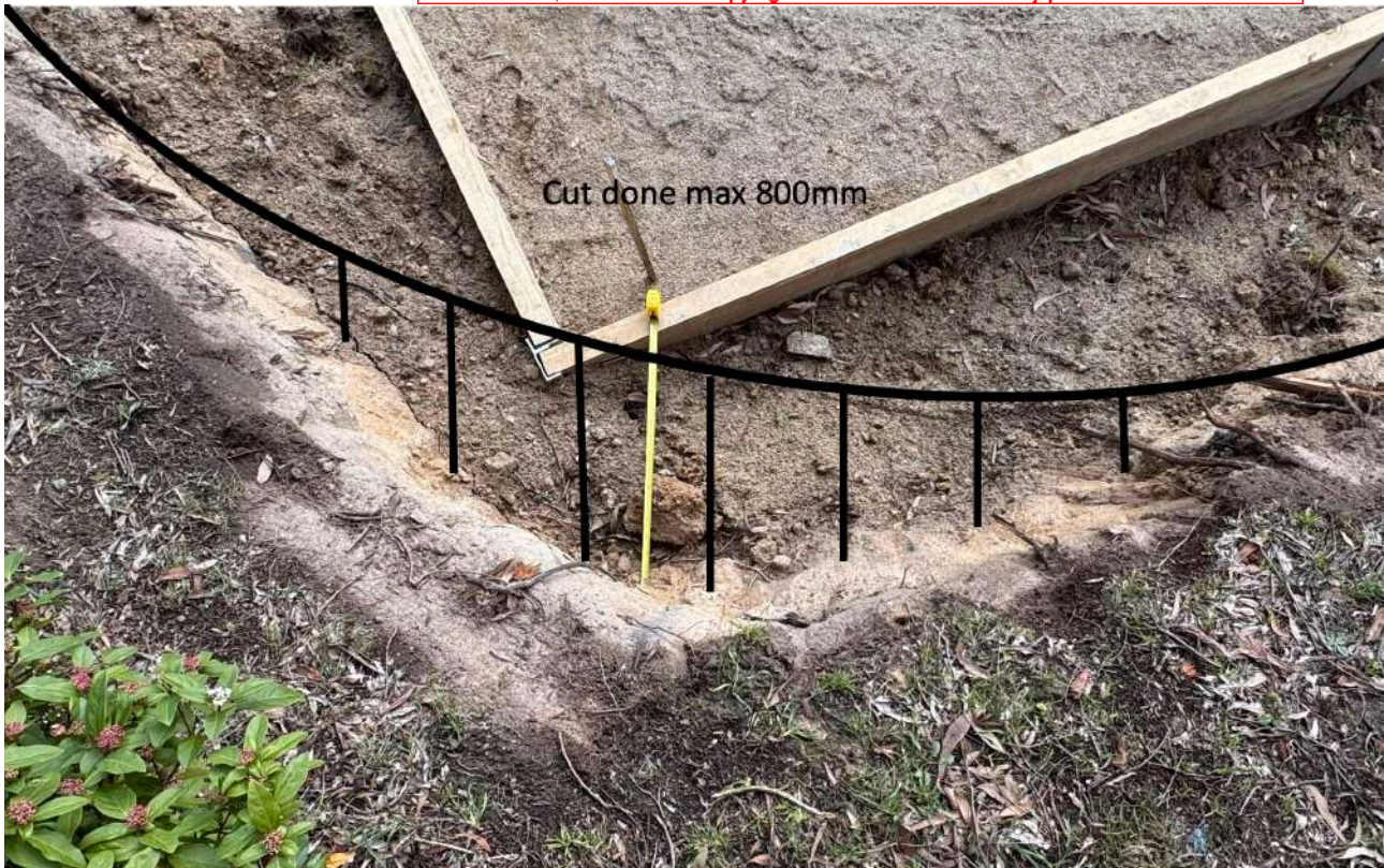
Aerial view showing the original cut (black curve) and the new cut made to accomodate the corner roof post.
