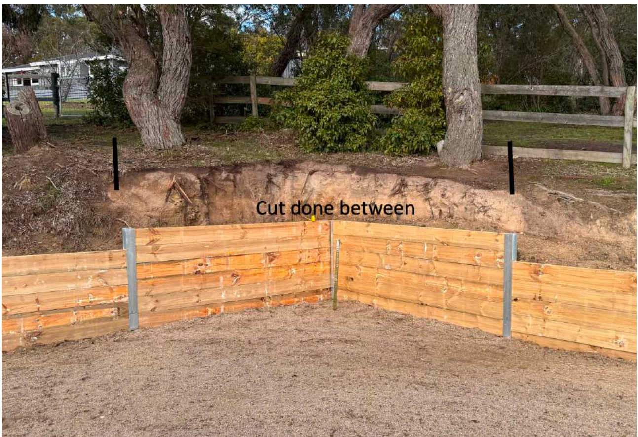
Showing the original cut and the new cut made to accomodate the corner roof post.
