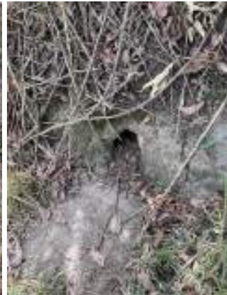
Soil profile in dam embankment – old rabbit warren
