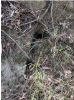
Soil profile in dam embankment – old rabbit warren
