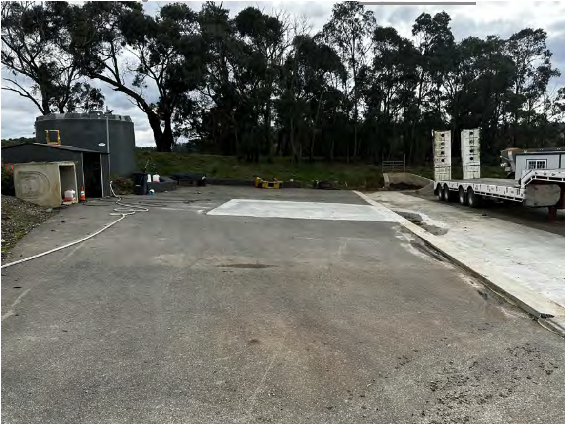
EXISTING WASH BAY - BITUMEN AND CONCRETE DRAINING TO CONCRETE DRAIN
