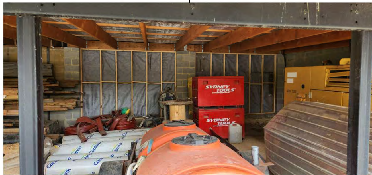
EXISTING TIMBER FRAMED INFILL WALL
