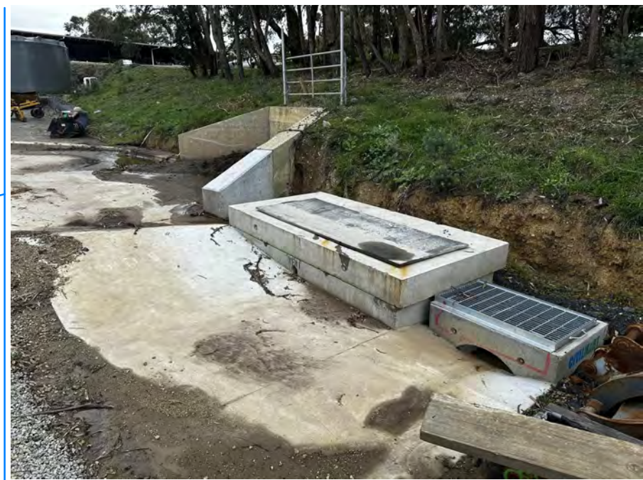
EXISTING TRIPPLE INTERCEPTOR
