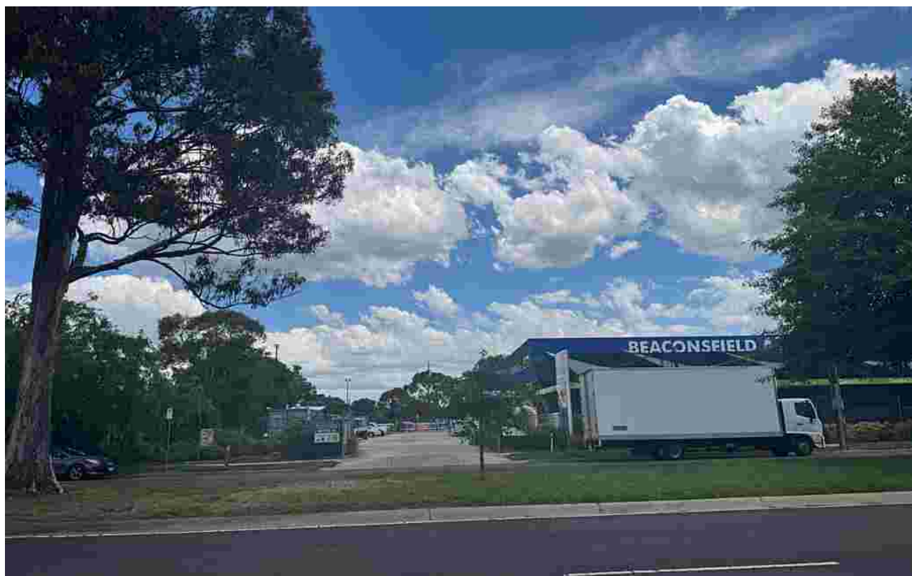
Figure 15: View south from the subject site – Old Princes Hwy (Taken by TB, December 2024)
