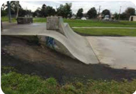
Existing batters worn exposing edge of ramps
