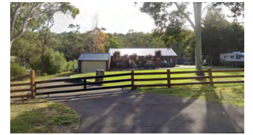
1 SUBJECT SITE: 12 FRASER AVENUE - EXISTING SINGLE STOREY DWELLING (BRICK VENEER)
