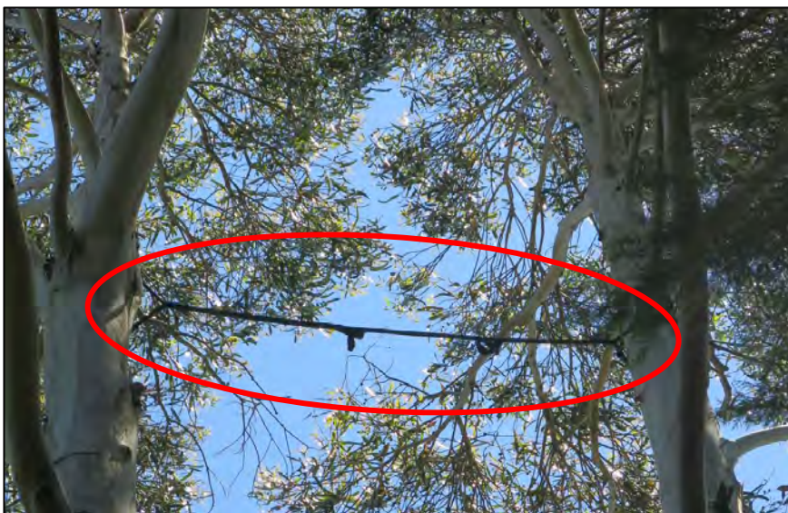
Figure 1 - Example of dynamic cable brace installed between tree components.
