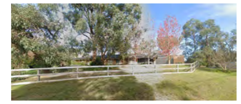
4 OPPOSITE SITE: 7 FRASER AVENUE - EXISTING SINGLE STOREY DWELLING (BRICK VENEER)
