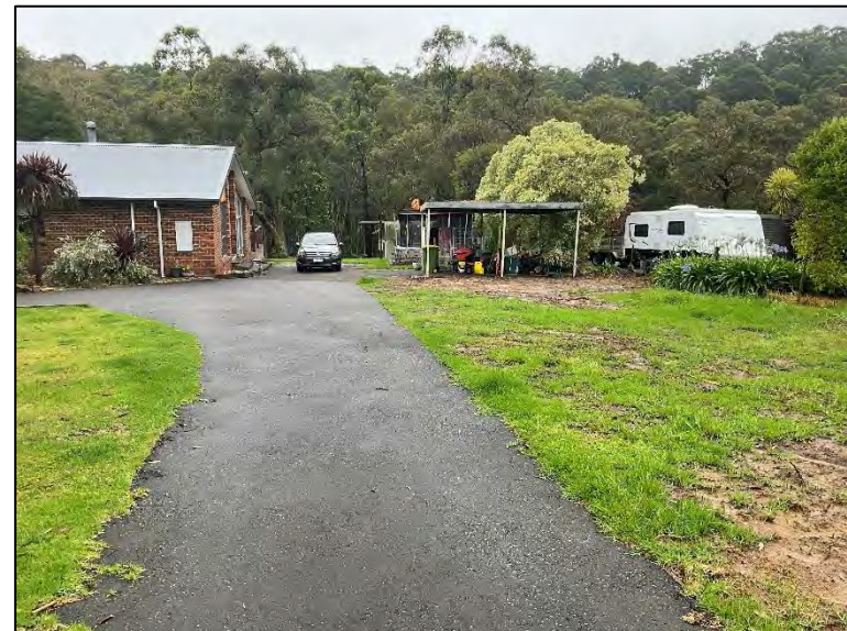
EXISTING DRIVEWAY VIEWED FROM THE NORTH
