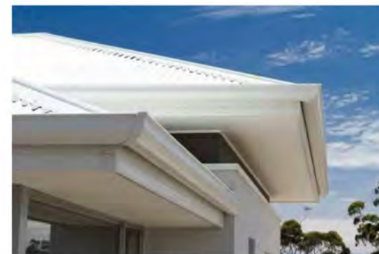
RFA-01 FASCIA: Pressed Metal - Colorbond Steel 'Surfmist' or similar
