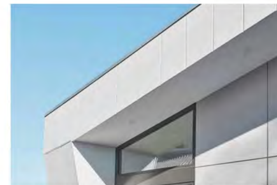
MTX-01 METAL CLADDING: JAMES HARDIE - 'Matrix Cladding' Profile or similar - Powdercoated Colorbond Steel 'Surfmist' or similar
