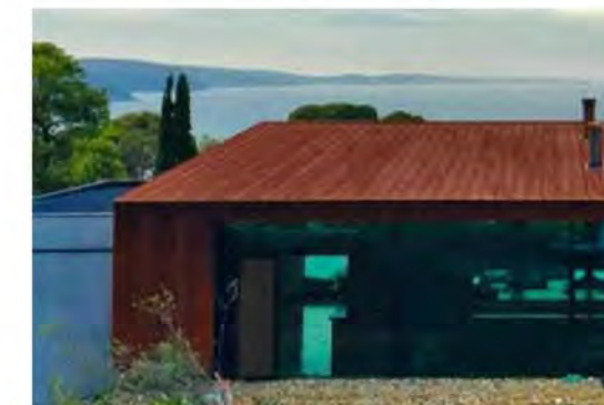
RSH-02 ROOF SHEETING: 'Interlocking Panel' Profile or similar - Pressed Metal - 'NEXTEEL - Weathering Steel (Corten) or similar
