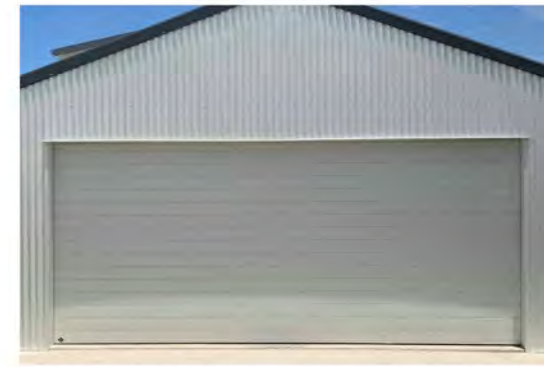
GAR-01 GARAGE DOOR: Powdercoated - Colorbond Steel 'Surfmist' or similar
