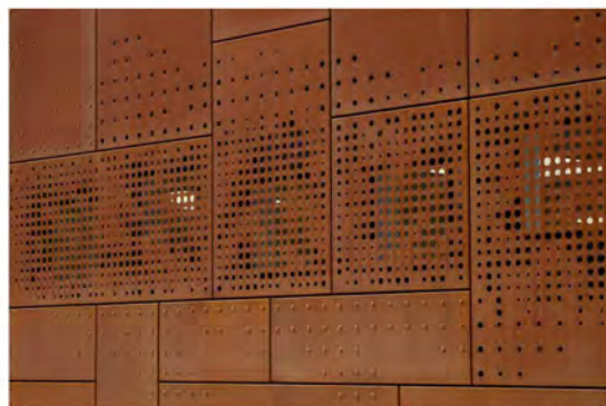
CLM-03 METAL CLADDING: Corten or similar - Perforated Corten Steel Sheet Panel or similar
