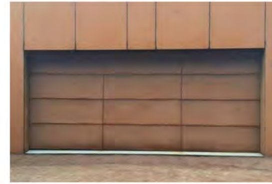
GAR-02 GARAGE DOOR: Powdercoated - Colorbond Steel 'Terrain' or similar
