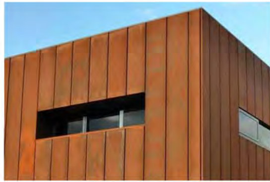
CLM-02 METAL CLADDING: Vertical - 'Interlocking Panel' Cladding Profile or similar - 'NEXTEEL - Weathering Steel (Corten) or similar
