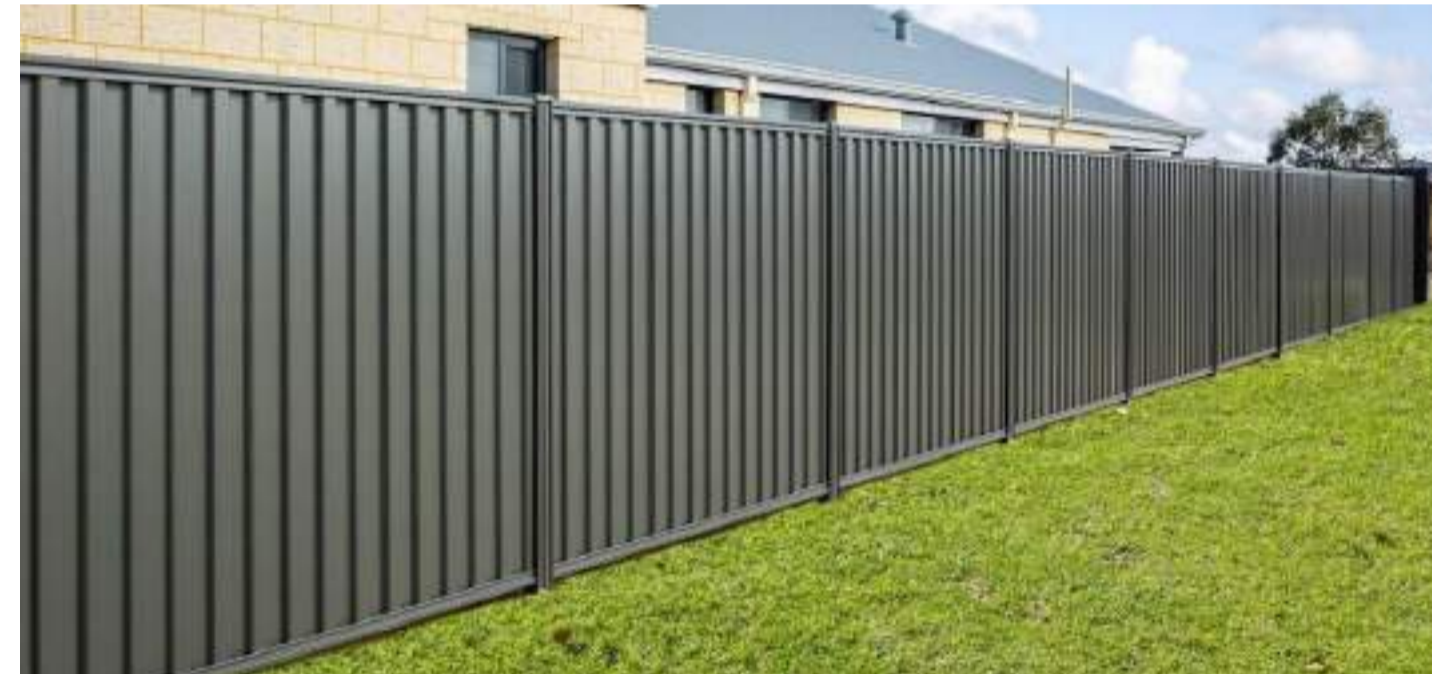
Fence Type A - Colorbond Fence - 1800mm high NOT TO SCALE
