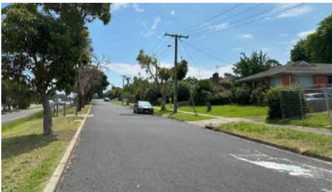
FIGURE 5: VIEW OF PRINCES HIGHWAY SERVICE ROAD FACING WEST
