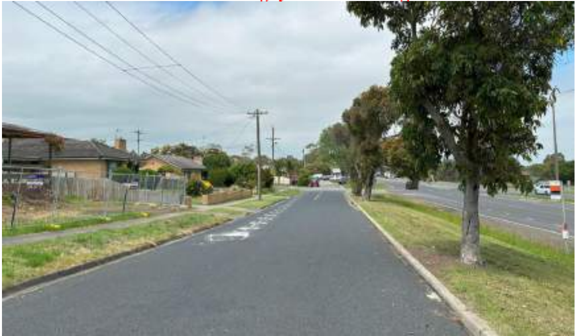
FIGURE 6: VIEW OF PRINCES HIGHWAY SERVICE ROAD FACING EAST
