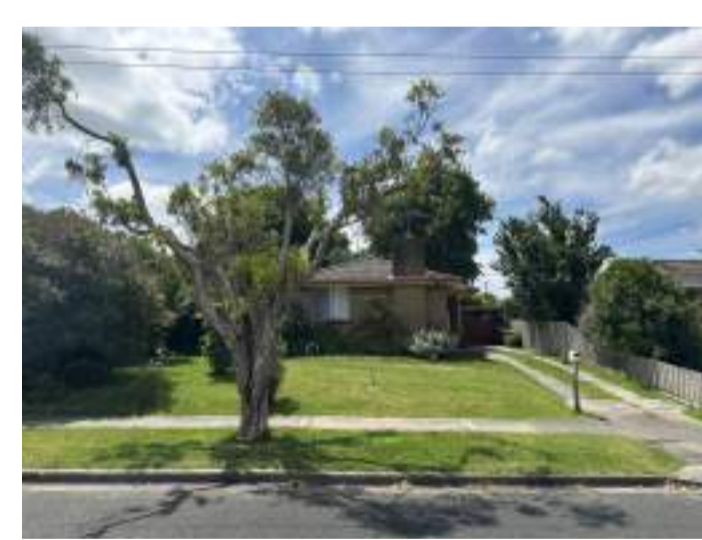
Photo #01 LOOKING NORTH AT NO.24 PRINCES HIGHWAY.
