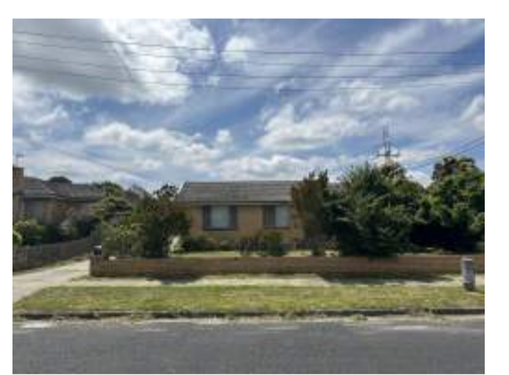
Photo #05 LOOKING NORTH AT NO.16 PRINCES HIGHWAY, CORNER ATKINS ROAD.
