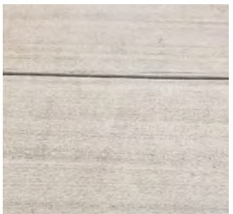
Exterior concrete paving – Broom Finish
