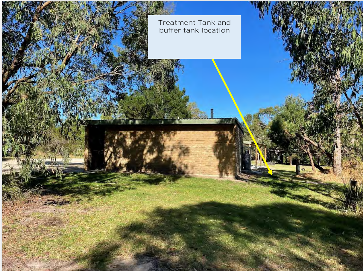
P3 - View towards the west depicting the existing toilet block (locked weekdays) and location of the proposed secondary treatment tank and buffer tank location (Garfield North Road, Garfield North).
