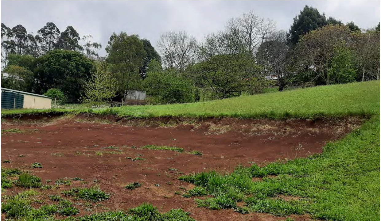
IMAGE 10 – Location of Building Envelope with existing site cut. View to the north west of the site.
