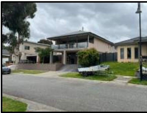
Figure 7: The front of the residential property at 5 Carey Street to the south of 7 Carey Crescent.
