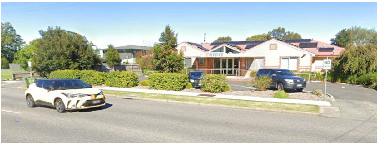
Figure 3: View looking west towards 5-7 Main Street site frontage
