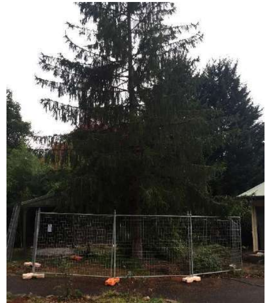
Figure 5.1. Tree protection fencing installed around a Norway Spruce
