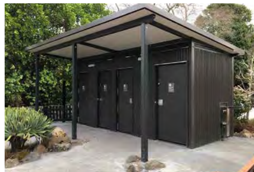
DDA compliant toilet unit with unisex, ambulant and disabled cubicles. Consider Colorbond cladding or similar that blends into the environment
