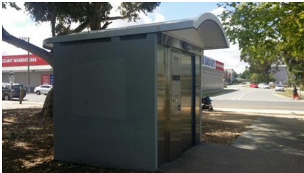
109089 Pakenham Bourke Park Exeloo
