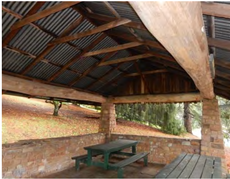
Internal view of Lakeside shelter showing roof framing. Note vertical boards to gable end.
