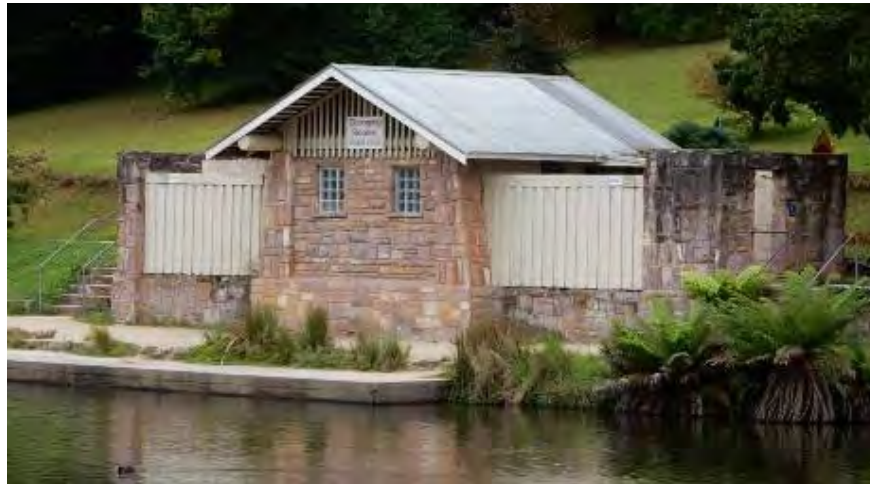
Lake Treganowan toilet block on the north-western side of the lake.
