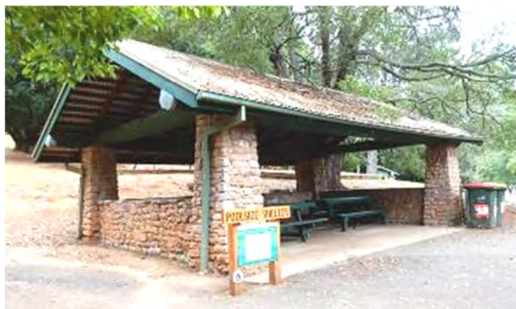
View of Poolside shelter from south-east. Note steel caps to ends of beams.
