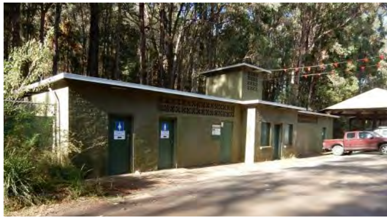
Maintenance building and Lion's Den toilets. The Lion's Den rotunda is to the right of the image.
