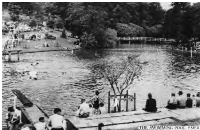
Southern end of Lake Treganowan with diving tower on the left, spring board in the foreground and timber bridge over Wattle Creek in the distance. This view was taken in front of the Lake Treganowan change rooms and toilet block.
