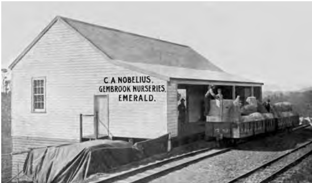
Packing Shed and siding 1904
