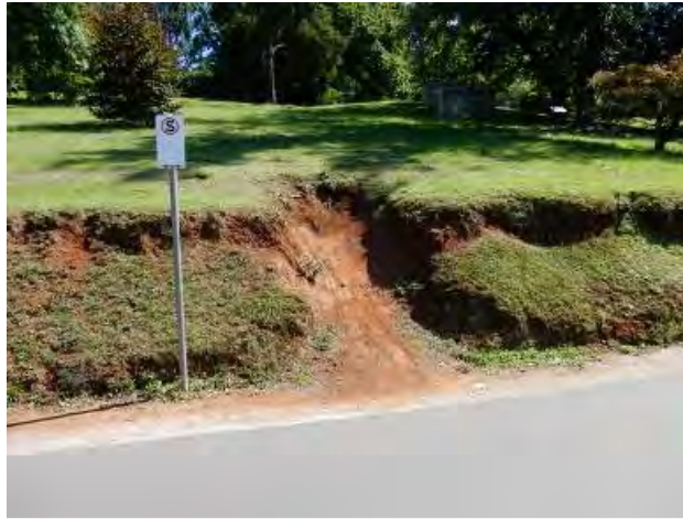
Track and embankment soil slump to Gus Ryberg arboretum off entry road.
