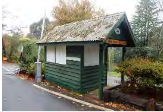
View of Ticket Box from the north.
